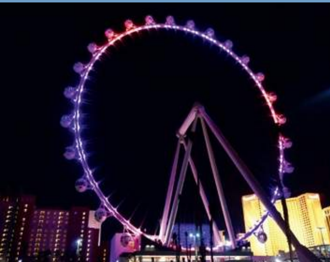
A High Roller with TMDs for Protection from Wind Forced Vibrations, Las Vegas, USA
