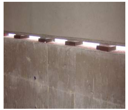
Wall on elastic pads
