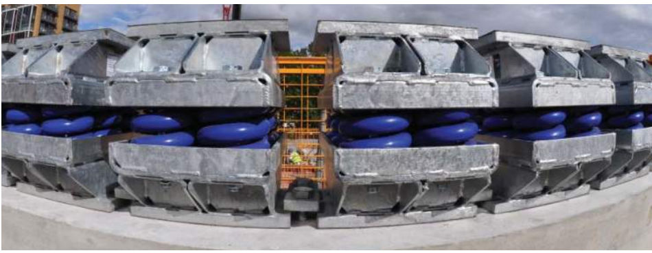
Pre-compressed spring isolators
