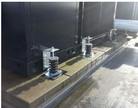
Adjustable spring mounts
