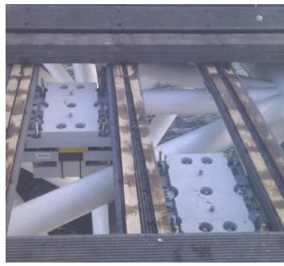
Installation under bridge
